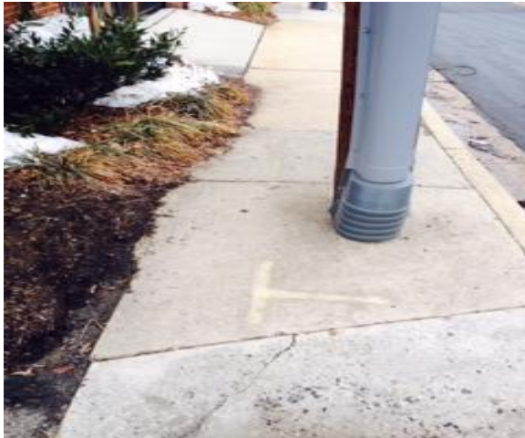
Older sidewalks blocked by utility poles, impassable for wheelchair or stroller use. Eg N Monroe St.
