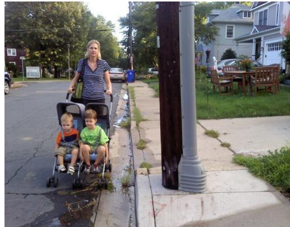
Older sidewalks blocked by utility poles, impassable for wheelchair or stroller use. Eg N Monroe St.
